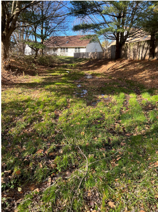
Pooled water unable to drain to roadway ditch.
